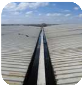
Over 600 linear meters of GRP valley gutter sealed with 551 ER Membrane
