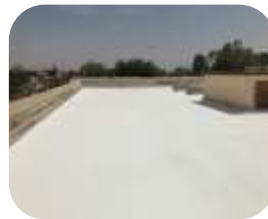
3000m 2 flat concrete roof coated with 2 x coats of 550 WR Membrane
