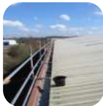
Over 600 linear meters of GRP valley gutter sealed with 551 ER Membrane
