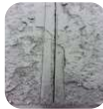
Mineral felt roof with leaking joints sealed with 2 x coats of 554 RB Membrane
