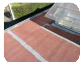
Leaking seams on a mineral felt roof sealed using 551 ER Membrane
