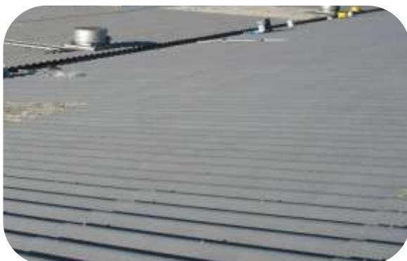
Metal roof primed with 506 Aluprime and coated with 550 WR Membrane
